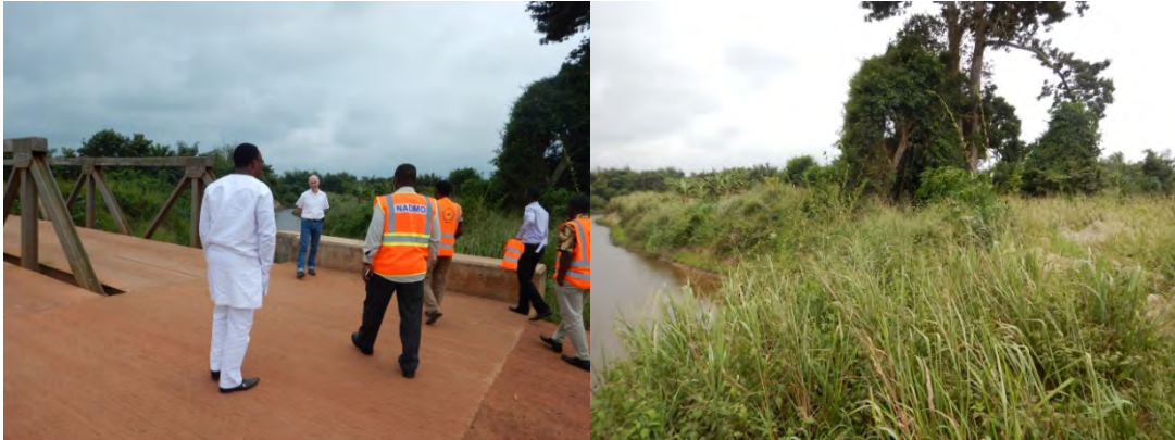
Figure 14. Upstream of bridge (stop 1) – the place where the river was dredged. Sediment was used to strengthen the river bank.
