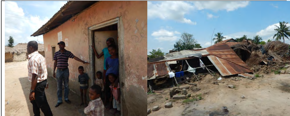
Figure 55: Resident indicates flood level (left), visible damage in the village due to flooding (right)
