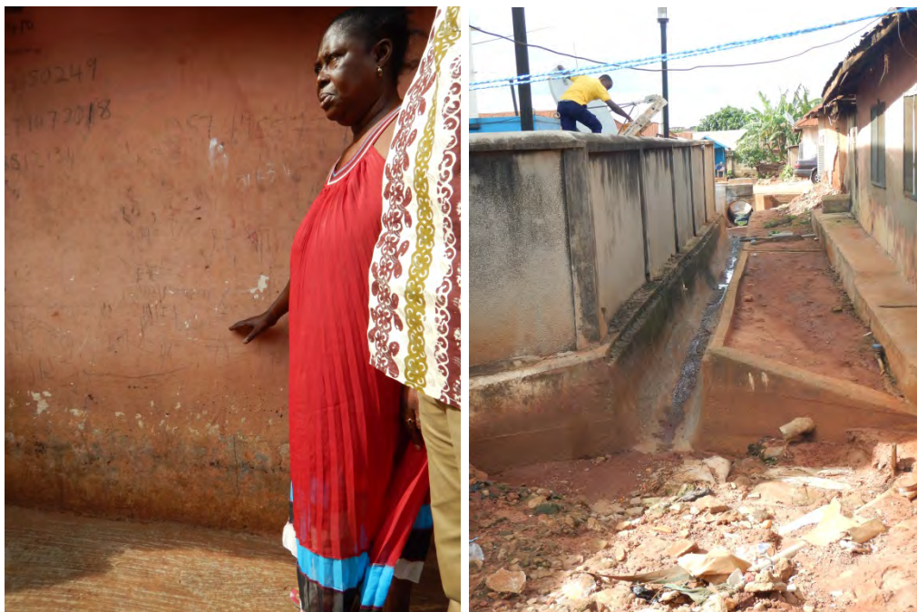
Figure 8. Ahenbronose: indication of flooding level (left) and lined outflow channel (right)
