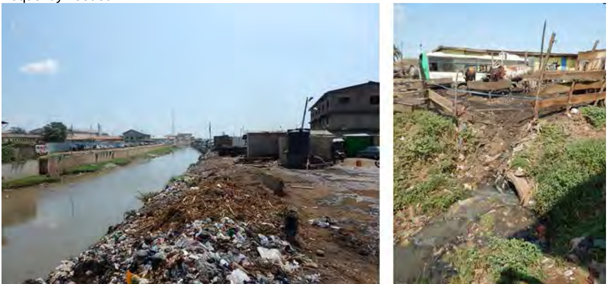
Figure 30: Odaw drain and local drain flowing into Odaw drain
