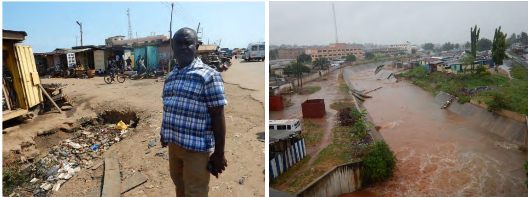
Figure 34: Examples of waste deposits in the Odaw catchment (left Avenor) and bad maintenance of the Odaw drain (right south Alogboshie)
