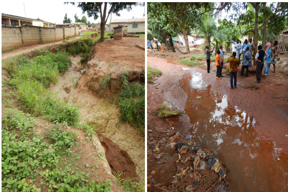
Figure 7. New Onyinase: images of the drainage channel
