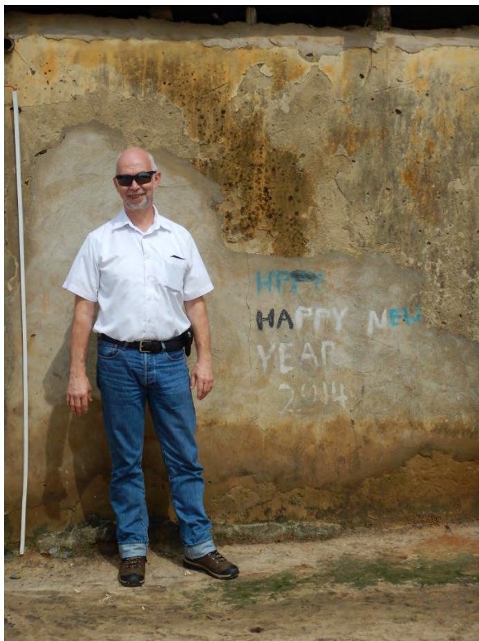
Figure 63. Flood level indication – recent flood level was at the height of the writing ‘Happy’
