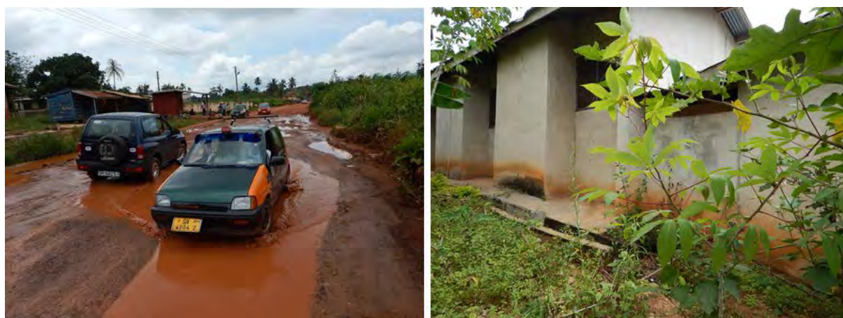
Figure 21: Begoro: flood marks
