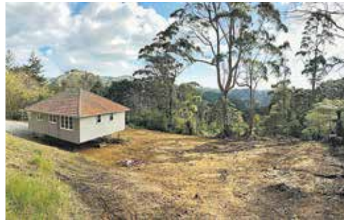
Relocated...One of the Hillary houses moving onto its new site in Swanson, west Auckland.
