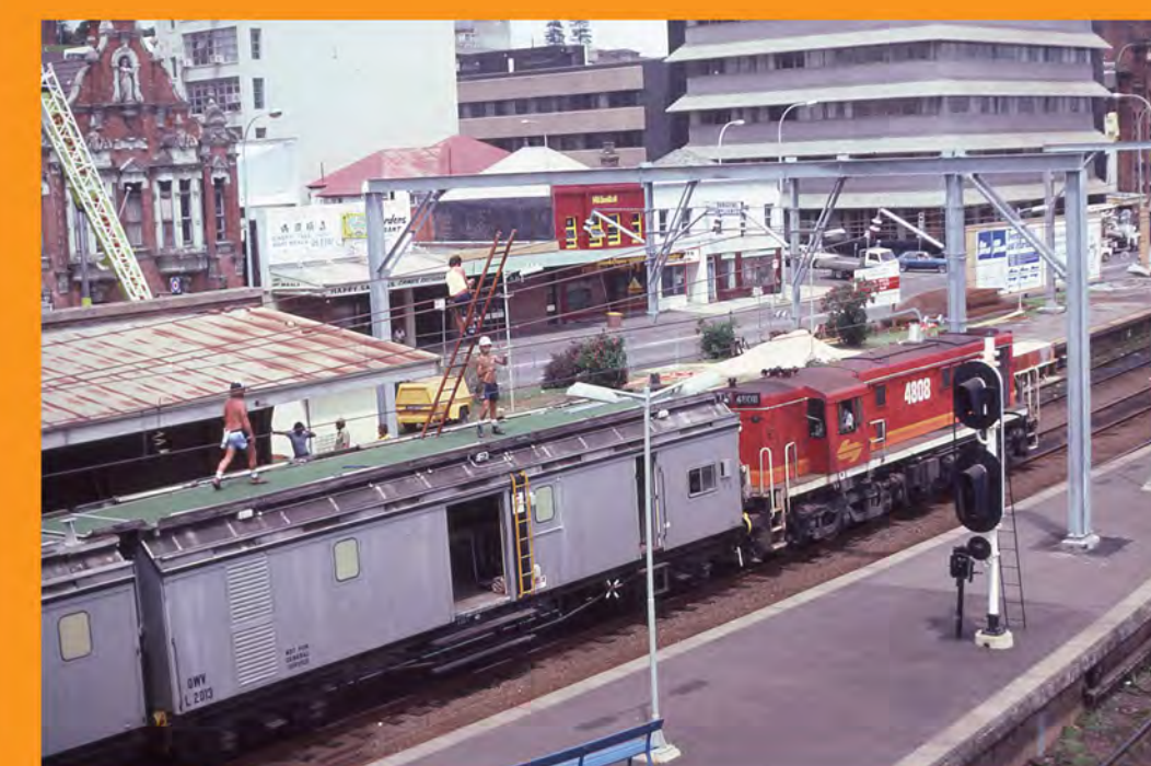
Above: Diesel-electric locomotive 4808 with workers on top of a wiring train, installing electrics at Newcastle Station on 14 November 1983. Courtesy of Ed Tonks.
