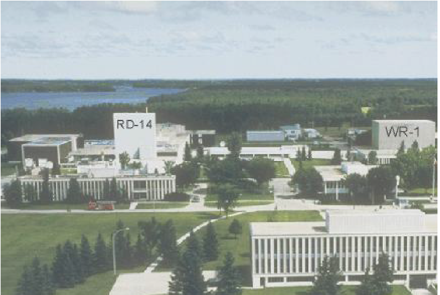
Photo: Whiteshell Nuclear Reactor 1 (cns-snc.ca)
