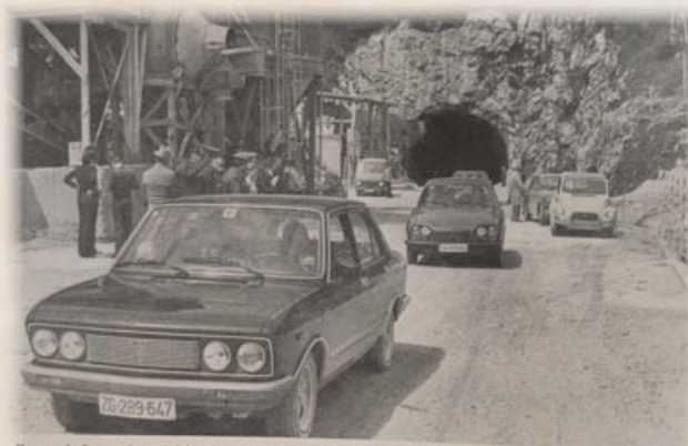
These are the first cars that passed through the Tunnel of Učka. When it will be completed, 1800 cars per hour will pass through.
