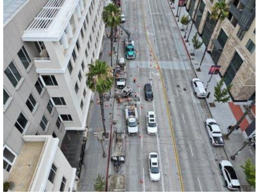
During summer 2025, crews successfully completed utility exploration along the alignment
