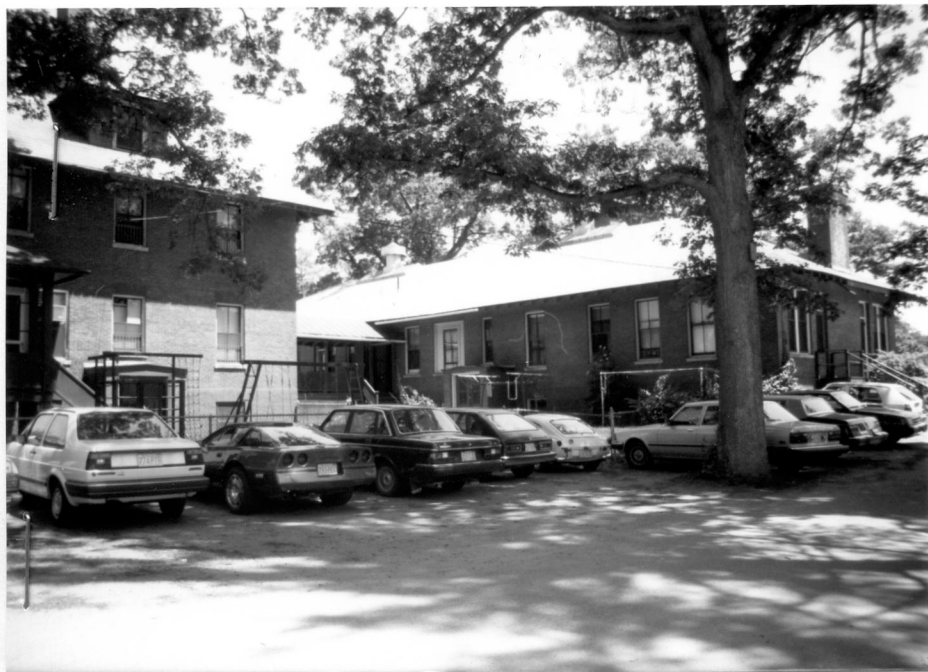
Newton Cottage Hospital: Contagious Wards
