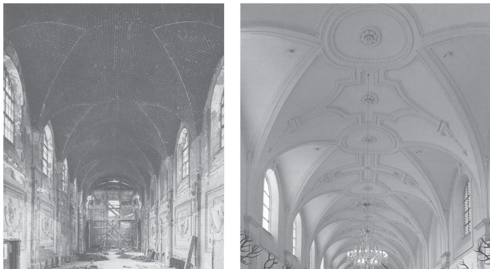
Figure 16. Old church of S. Agustin, now the German Hunting and Fishing Museum, in Munich. Left: Main vault reconstructed with tile vaults just after completion (Rank 1962), see also plate XXII; right: The vault in its finished state (Basiner et al. 2012, 366).
