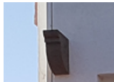
Decorative Exposed Rafter Tails
