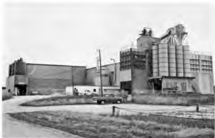
Figure 6. High-silica sand processing plant, Indiana Glass Sand Co., Elizabeth, Harrison County.
