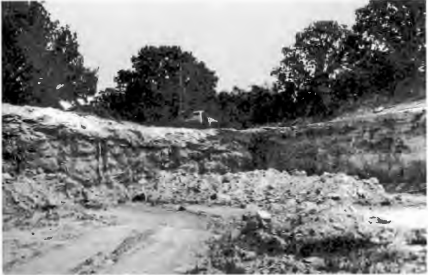
Figure 5. Sandstones of the Mansfield Formation exposed in the Harrison Steel Co. quarry about 1 mile southwest of Attica in the NW¼SE¼ sec. 13, T. 21 N., R. 8 W., Fountain County. These sandstones are crushed and used for molding sand.
