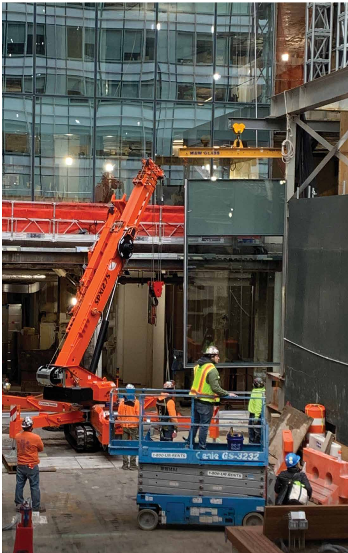
Above W&W Glass uses a hydraulic actuator to test the curtain wall anchor assembly fastened into the floor slab for combined tension/shear load. In some areas, a new slab structure was attached for strength reinforcement of the original structure. Left and facing Installation of the curtain wall by W&W Glass. Facing, renderings Details of the facade's slender mullions.
