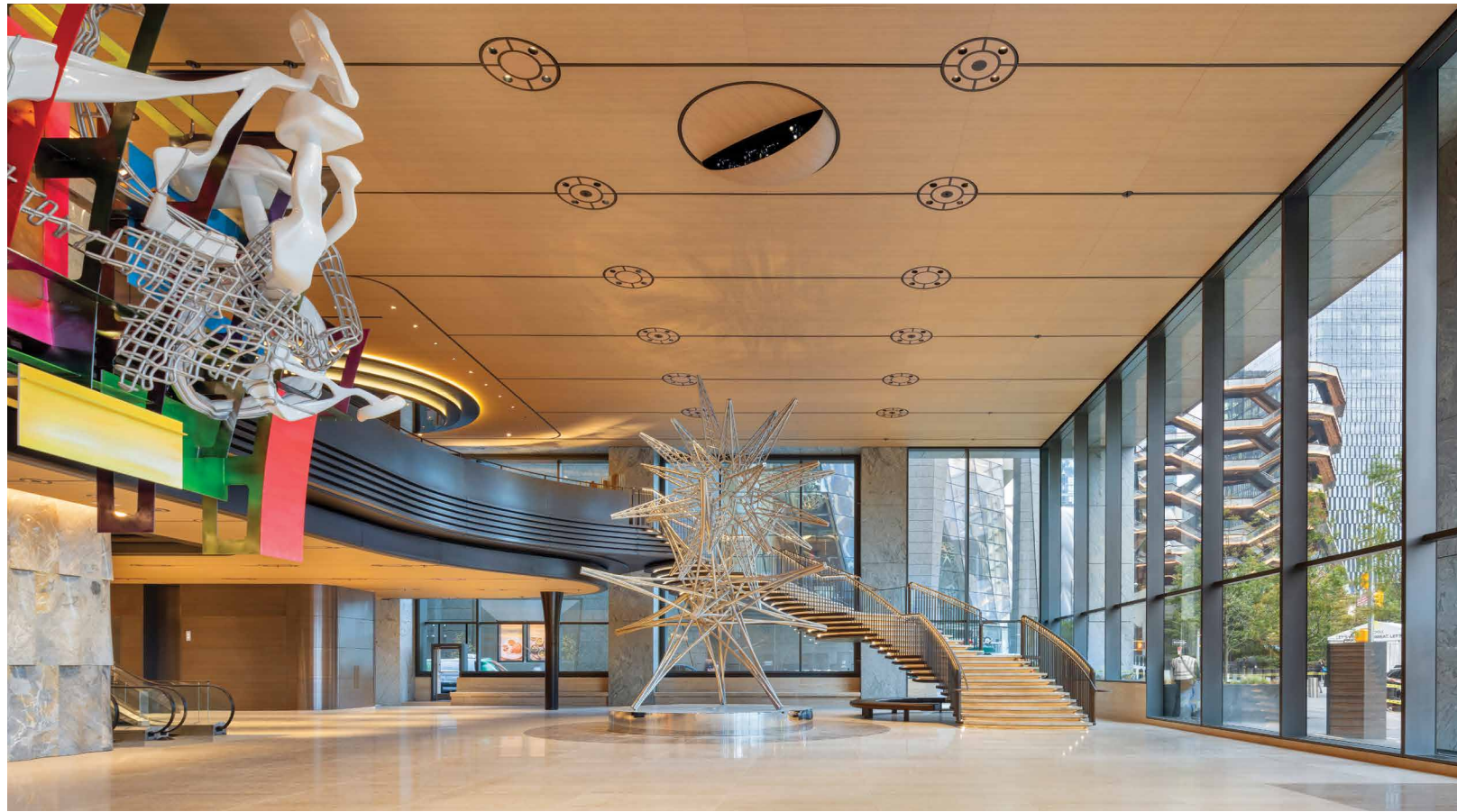
Above In addition to steel, the stair features aluminum trims and a bronze patina. It was assembled on-site by a crew of ironworkers from Local 580, employed by installation contractor Monumental, Inc. Facing page The stair under construction in 2021.
