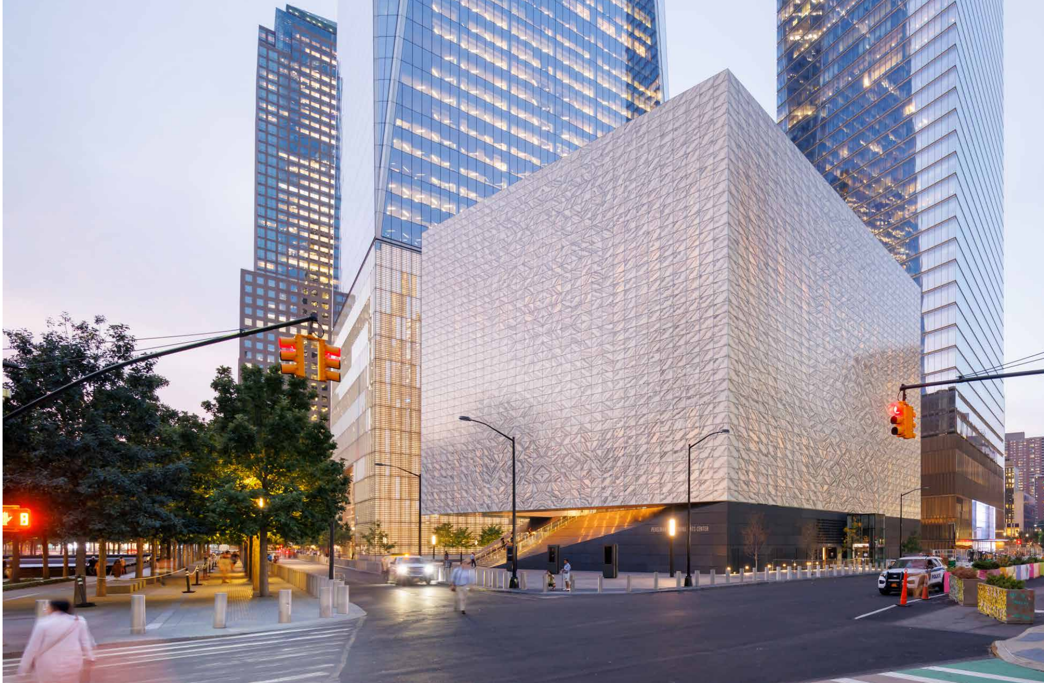
Above The facade’s marble was book-matched to create a biaxially symmetric pattern that is identical on all four sides of the building. It allows sunlight to radiate in during the day and project a glow from within at night. Left, top An interior corridor on the theater level. Left, bottom The venue’s restaurant, Metropolis by Marcus Samuelsson, was designed by Rockwell Group.
