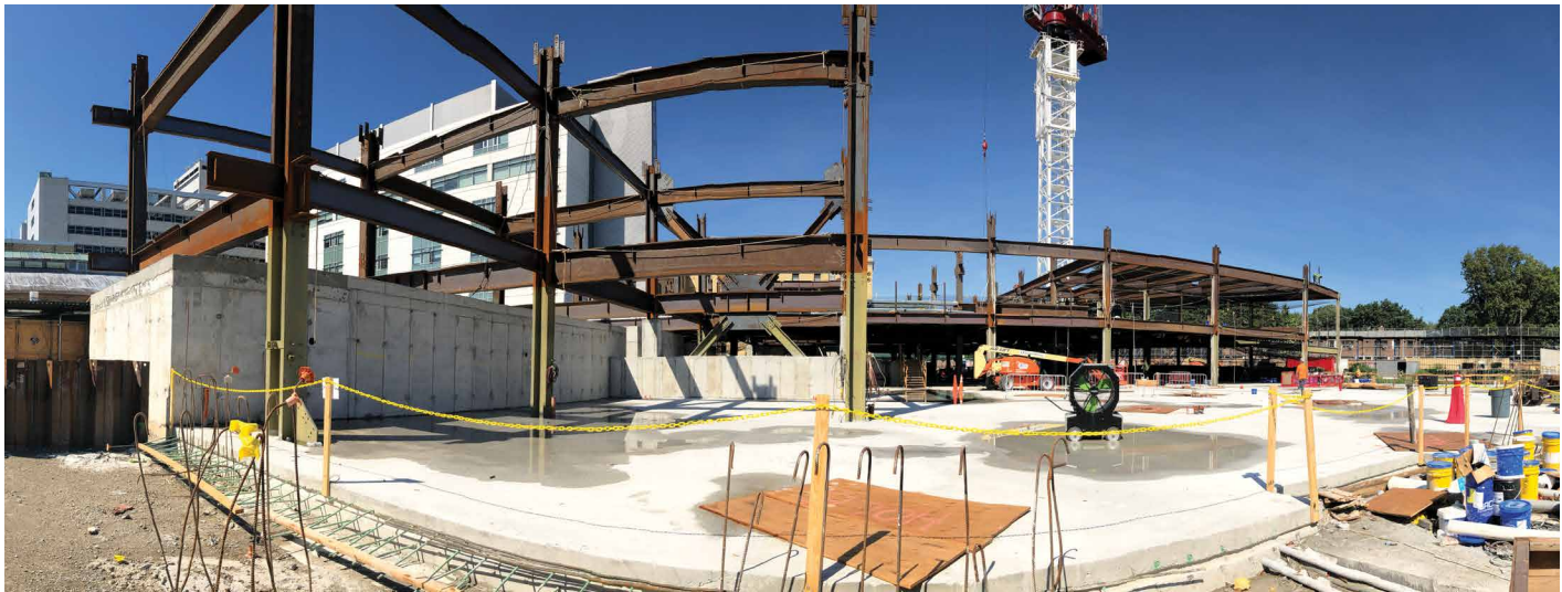
This page: Top and center: Courtesy Stonebridge Steel Erection. Bottom: Courtesy NBBJ
