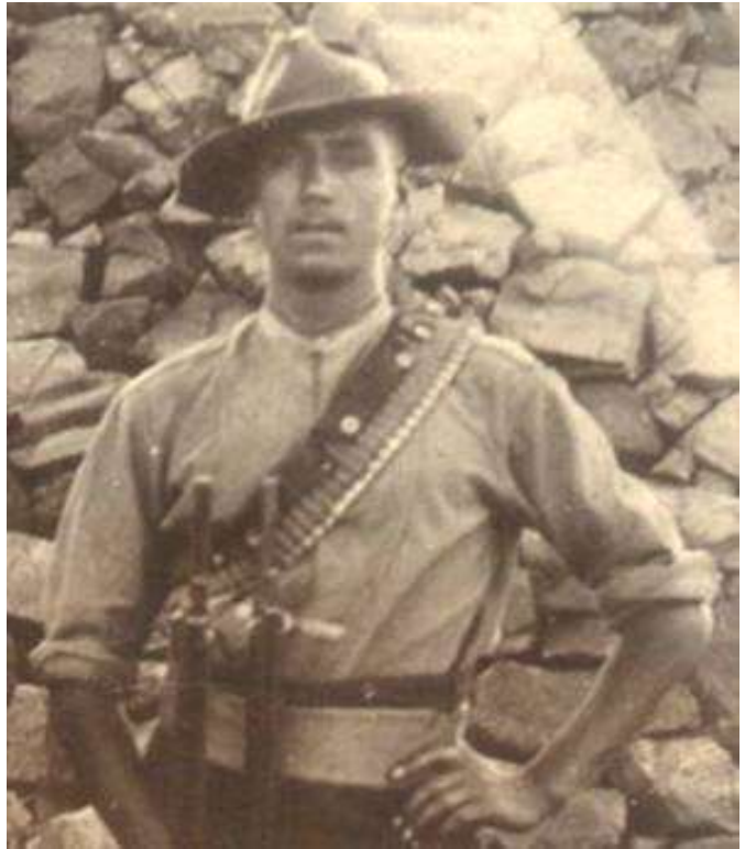
This blockhouse guard is wearing a disposable Mills emergency bandolier with flaps. Note the flimsy flaps and nail-on buttons.
