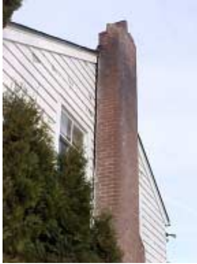
Figure 3.1.26 Separation and Failure of the Chimney of a Three-Story Wood Frame House in Olympia.
