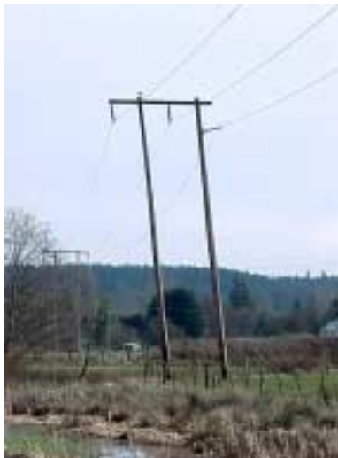
Figure 5.7.1 Permanent Lateral Drift of a Wood Electrical Pylon in the Epicentral Region of Nisqually Valley.
