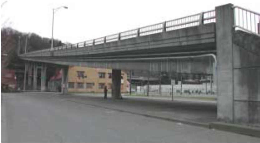
Figure 4.1.1 General View of Holgate Bridge.
