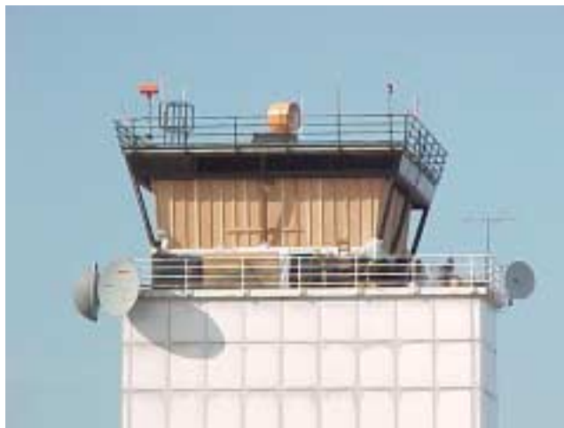
Figure 5.4.1 Control Tower Shattered Windows Boarded with Plywood at Sea-Tac Airport.
