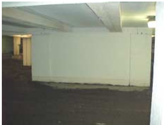
Figure 3.1.33 Added Reinforced Concrete Shear Walls in the Basement of the Cobalt Group Building in Downtown Seattle.
