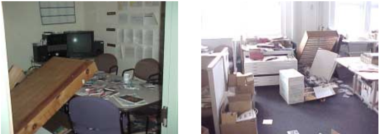
Figure 5.1.4 Damage Caused by Unanchored Furniture Items and Building Contents in Starbucks Headquarters in Seattle.
