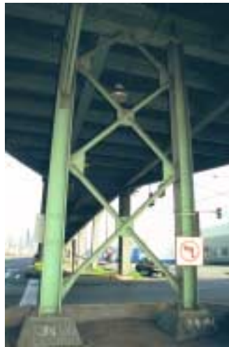
Figure 4.3.3 X-braced Steel Substructure.
