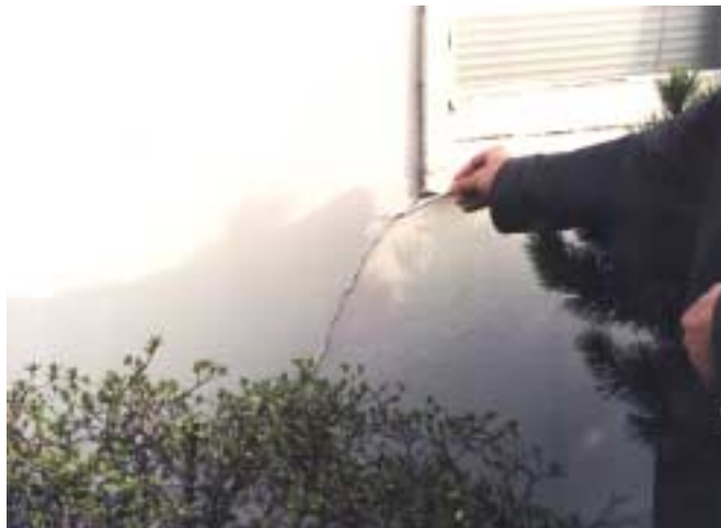
Figure 5.3.1 Diagonal Cracking of Stucco between Window Openings in a Three-Story Apartment Building in Olympia.
