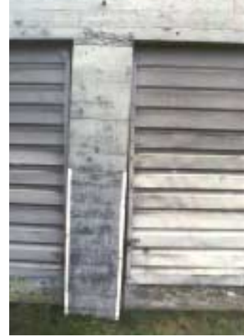
Figure 3.3.6 Cracking in Beam-to-Column Joints of a Concrete Garage Unit on Franklin Street in Olympia.
