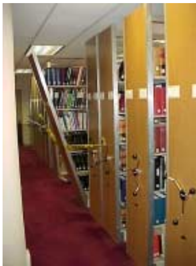
Figure 5.5.3 Undamaged Movable Compact Bookshelves and Leaning Conventional Bookshelves in the Main Library of the Temple of Justice Building in Olympia.
