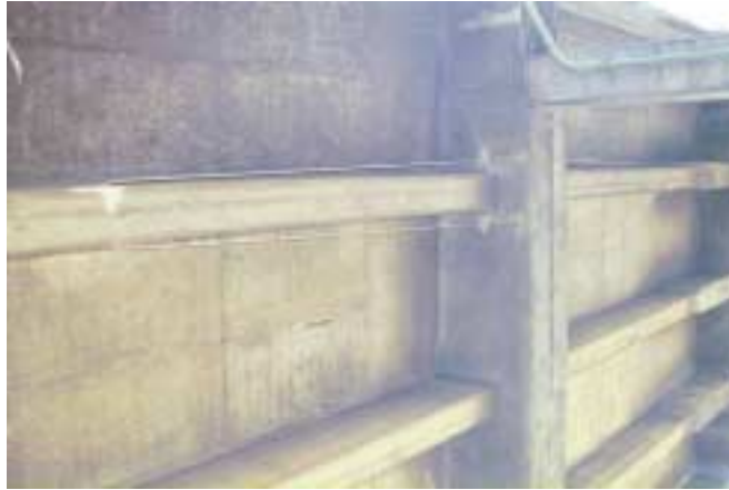
Figure 4.3.2 Cable Restrainers in Superstructures.
