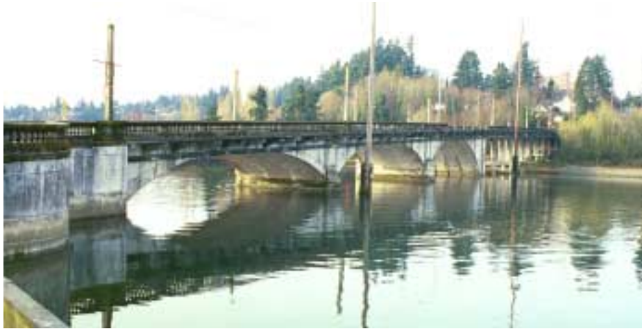
Figure 4.4.1 Global View of Fourth Avenue Bridge.
