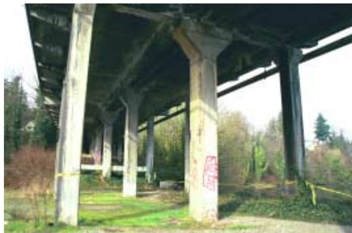
Figure 4.4.2 Bridge Bent Configuration.
