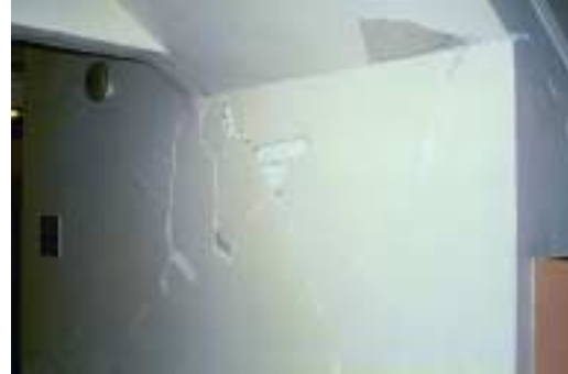
Figure 5.2.5 Cracking of Plastered Walls in the Stair Wells of the Olympian Apartments in Olympia.
