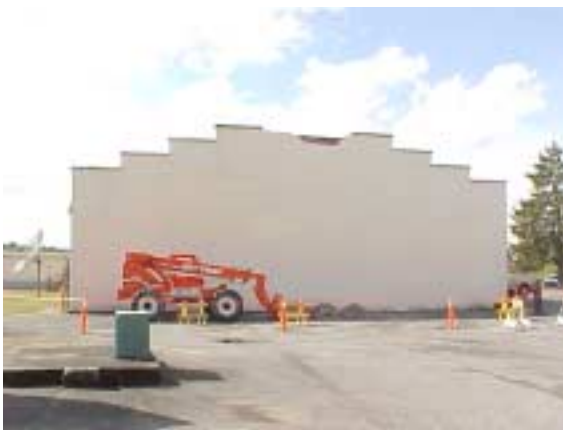
Figure 3.1.23 Failure of a Stepped Masonry Parapet in a Two-Story Military Dormitory Building in Fort Lewis.
