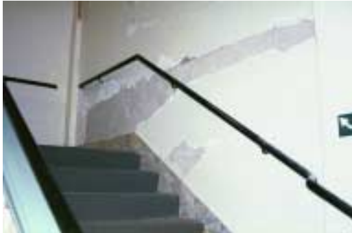
Figure 5.2.5 Cracking of Plastered Walls in the Stair Wells of the Olympian Apartments in Olympia.
