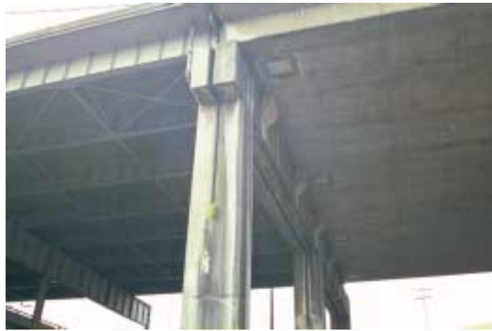
Figure 4.2.2 Bent 25 with Split Reinforced Concrete Columns.
