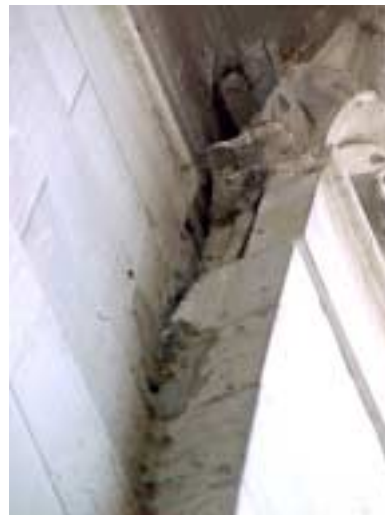
Figure 3.1.2 Severe Cracking of a Nonstructural Sandstone Pilaster at the Dome of the Legislative Building in Olympia.
