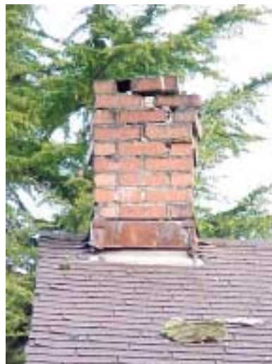
Figure 3.1.25 Chimney Failure in a Three-Story Wood Frame Apartment Building in Olympia.
