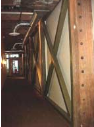
Figure 3.1.32 Diagonal Tubular Cross-Braces to Seismically Upgrade the Cobalt Group Building in Downtown Seattle.
