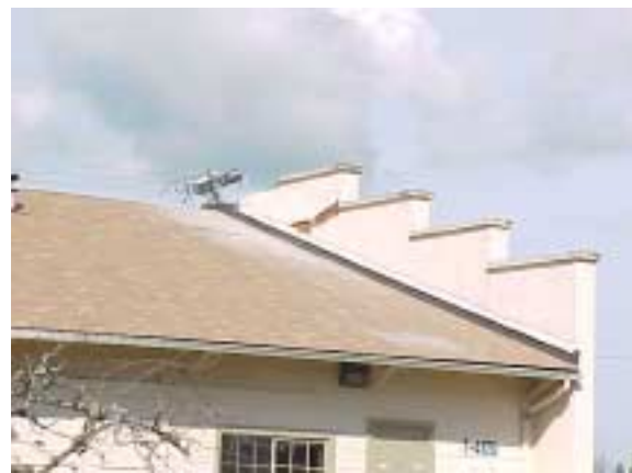
Figure 3.1.23 Failure of a Stepped Masonry Parapet in a Two-Story Military Dormitory Building in Fort Lewis.
