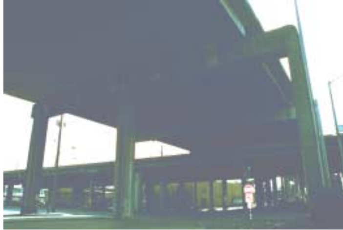
Figure 4.2.1 Spokane Bridge Overcross.
