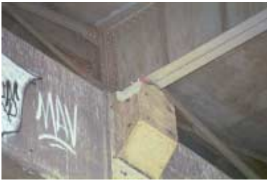
Figure 4.2.4 Damage to Catchers.
