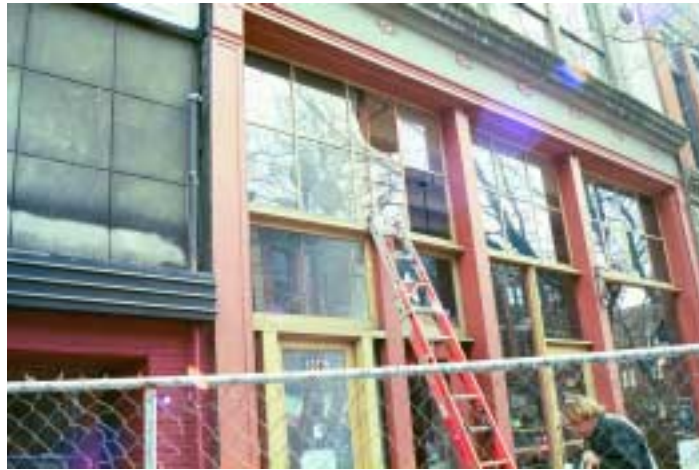
Figure 5.4.2 Replacing Broken Windowpanes in the Pioneer Square Area of Seattle.
