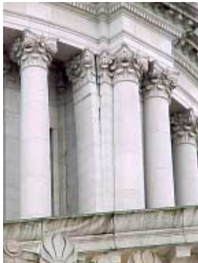
Figure 3.1.2 Severe Cracking of a Nonstructural Sandstone Pilaster at the Dome of the Legislative Building in Olympia.
