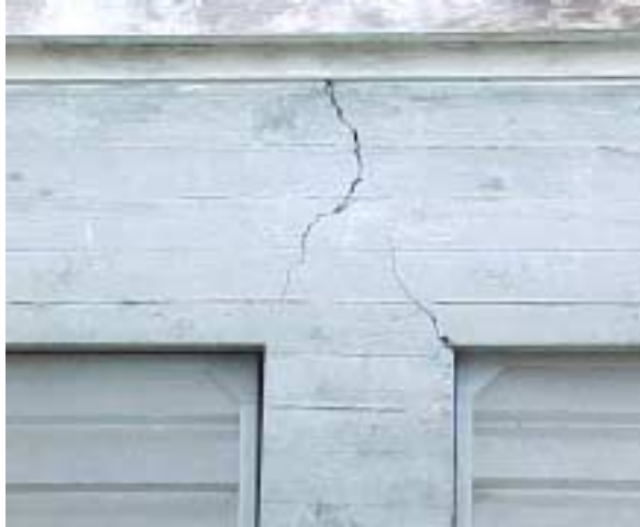
Figure 3.3.6 Cracking in Beam-to-Column Joints of a Concrete Garage Unit on Franklin Street in Olympia.
