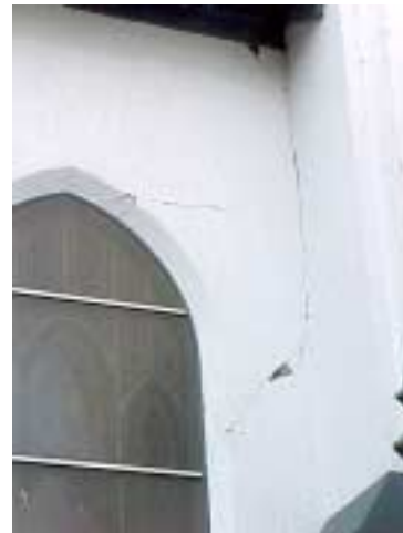
Figure 3.1.21 In-plane Cracking of Masonry Walls of the First Christian Church in Olympia.
