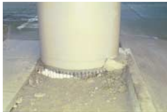
Figure 4.3.1 Steel Jacketed Reinforced Concrete Columns.
