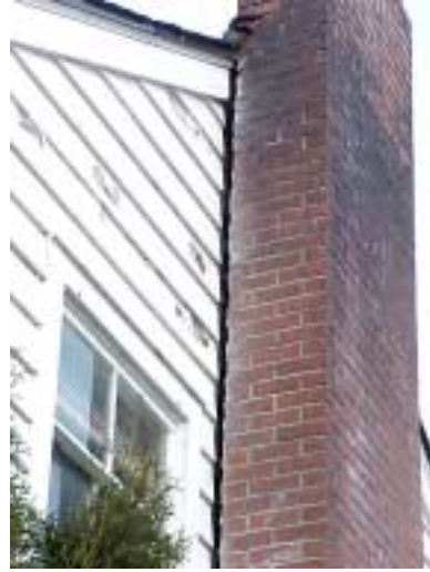
Figure 3.1.26 Separation and Failure of the Chimney of a Three-Story Wood Frame House in Olympia.
