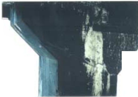
Figure 4.4.4 Bridge Column Condition in 1994 2 .
