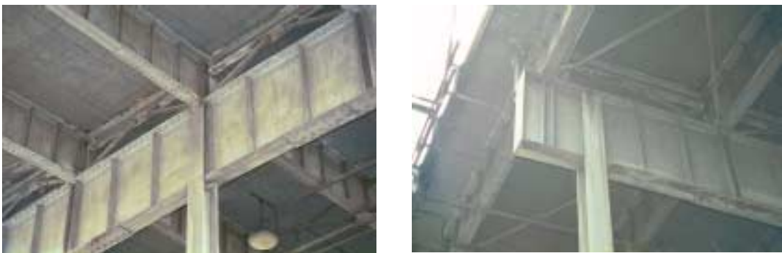
Figure 4.2.7 Bent 26 with Steel Substructures.
