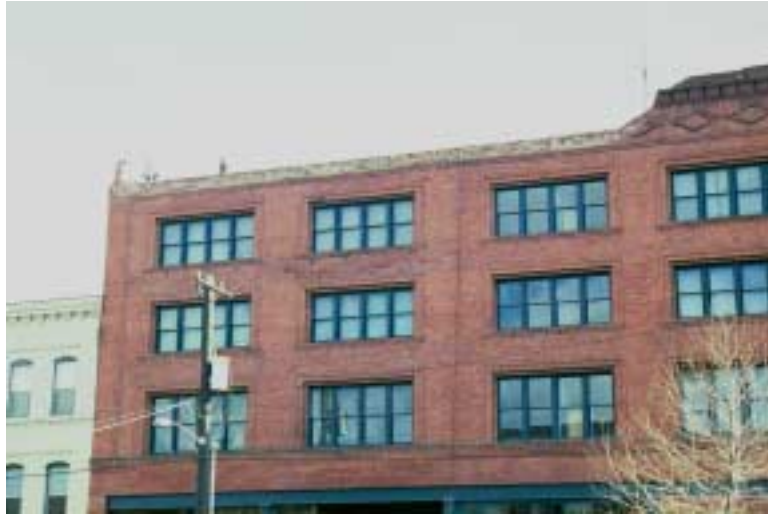
Figure 3.1.24 Collapse of an Unreinforced Parapet to the Building at 558 First Avenue South in Seattle.
