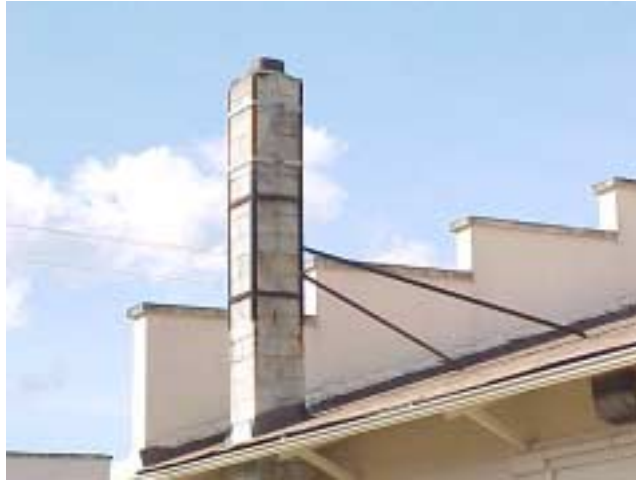
Figure 3.1.28 Undamaged Braced Chimney of a Wood Frame Army Barrack in Fort Lewis.
