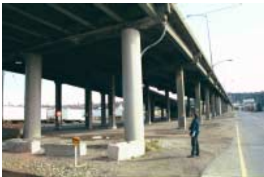
Figure 4.3.1 Steel Jacketed Reinforced Concrete Columns.
