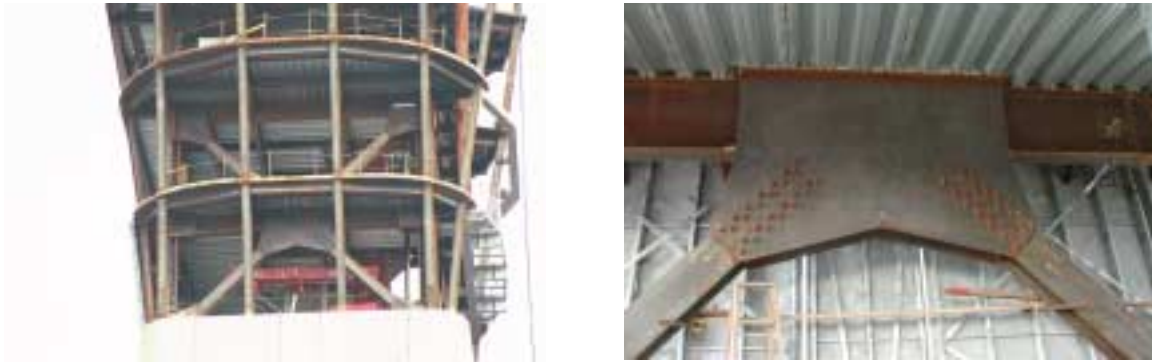
Figure 3.2.9 Super X-Braces for Special Concentrically Braced Frame.
