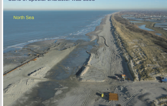
Construction: Beach and foreshore nourishment 2008/9 Sand of special character was used
