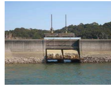
Opening the floodgate on the concrete dike
