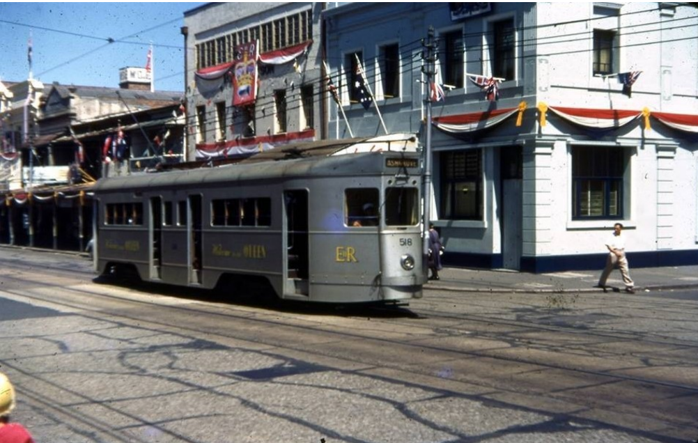
Below: A tram about to pass the Transcontinental Hotel along George Street.
