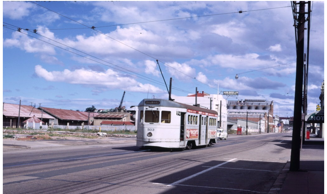
Above: A tram heads along Grey Street at South Brisbane.
