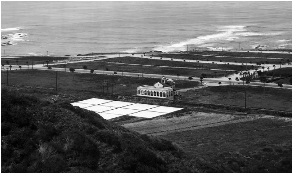
In 1926, the San Carlos Electric Railroad Station of the La Jolla and San Diego Electric line stood alone in the virtually undeveloped La Jolla Hermosa area. The San Carlos station was completed in 1924 and remained in service until 1940 when the "Last Car" took its last trip. The La Jolla United Methodist Church acquired the building in 1953 and, after extensive alterations, converted the former station into a home for its congregation. ©SDHS #9199.
