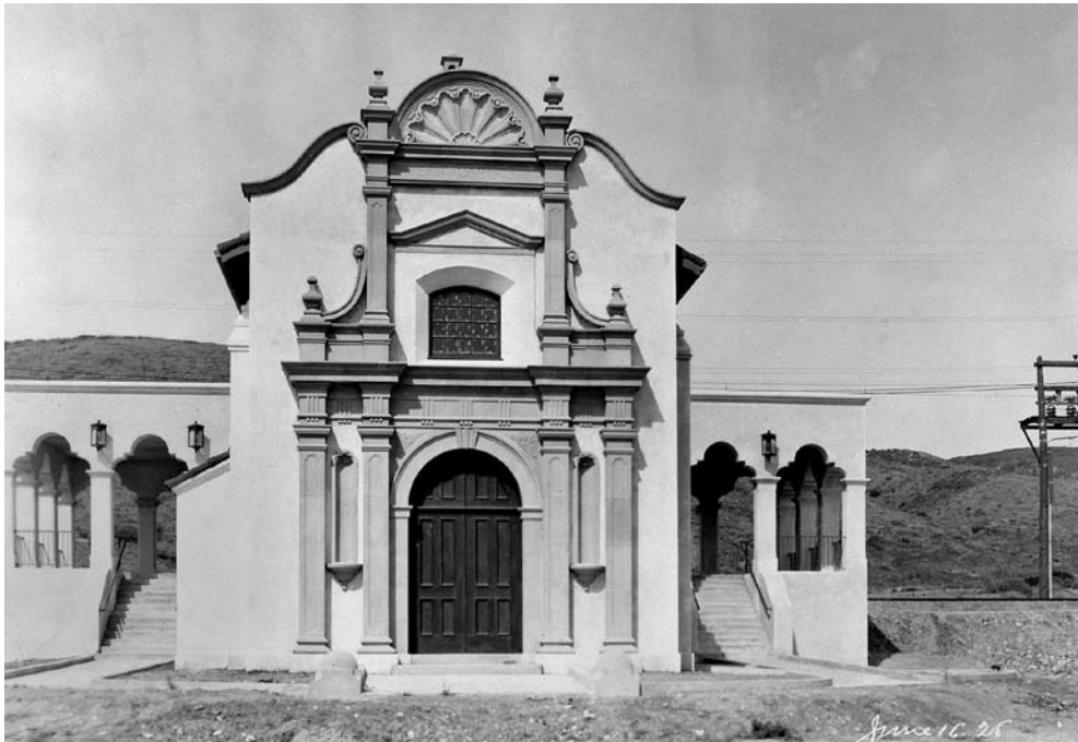
The San Diego Electric Railway named stations along the La Jolla and San Diego Electric line after California's missions, according to the December 12, 1924 edition of the La Jolla Journal. It adopted the Spanish Colonial architectural style for the San Carlos Electric Railway Station in La Jolla. In 1929, the railway planned an upscale restaurant for the San Carlos station with the intention of attracting locals and out-of-towners. ©SDHS #92:18728.
