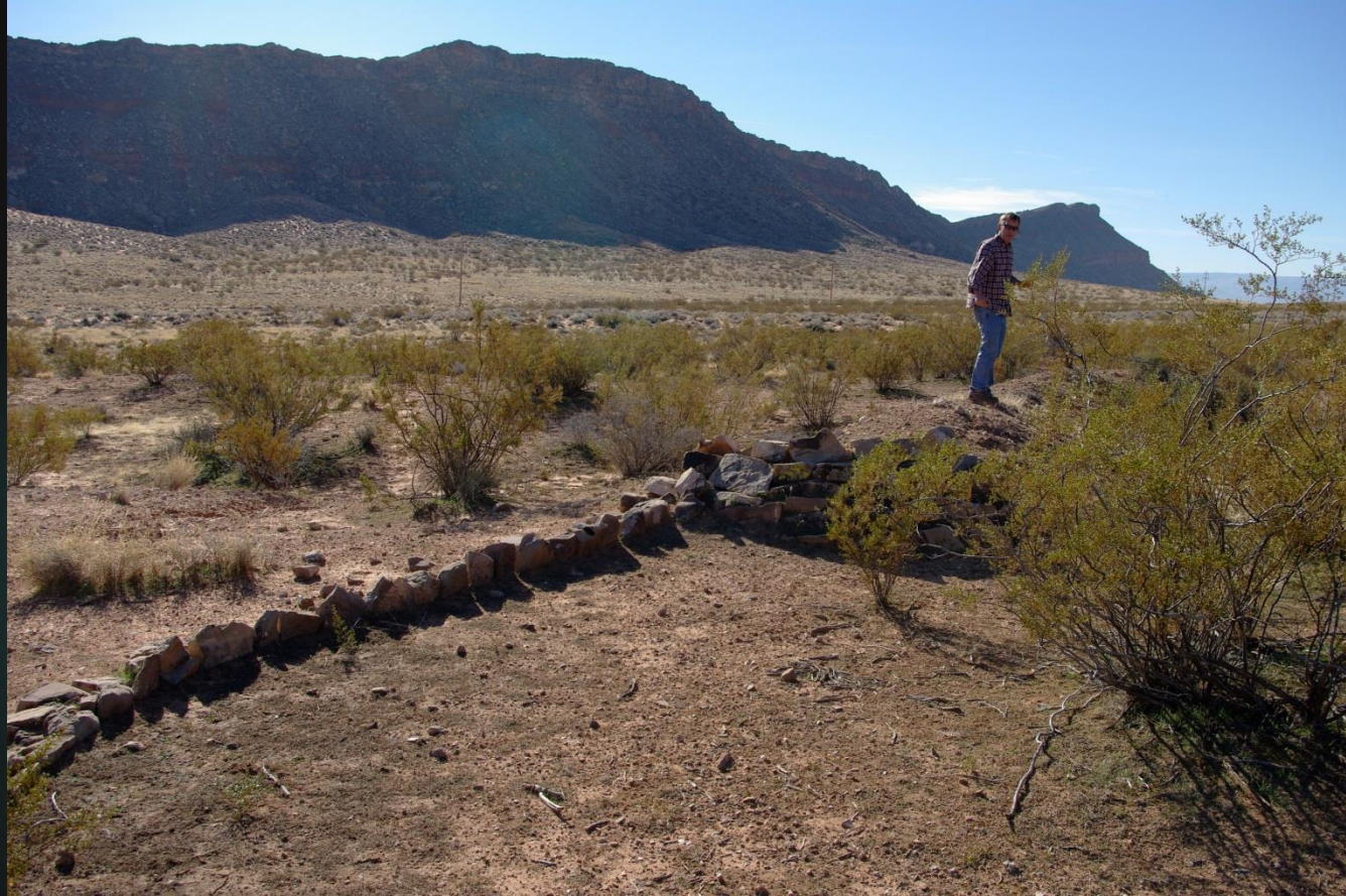
Earthen Berm and Rock Diversion Dam
