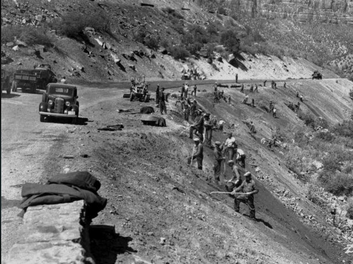
Shoring up Talus Slopes in Zion National Park. National Park Service Photo
