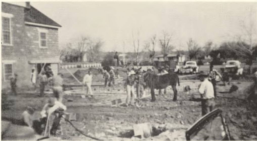
Beginning of Chapel Construction
