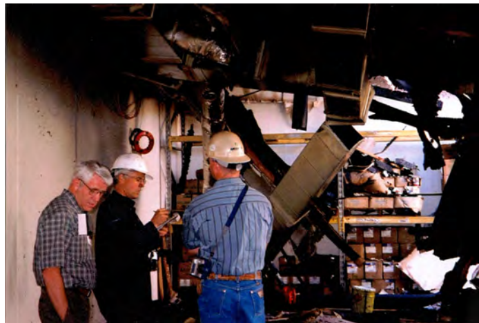
Cannery director Dale Hicken, a state inspector and a contractor assess damage to the cannery on April 30, 2003, following a fire on April 29 th .
