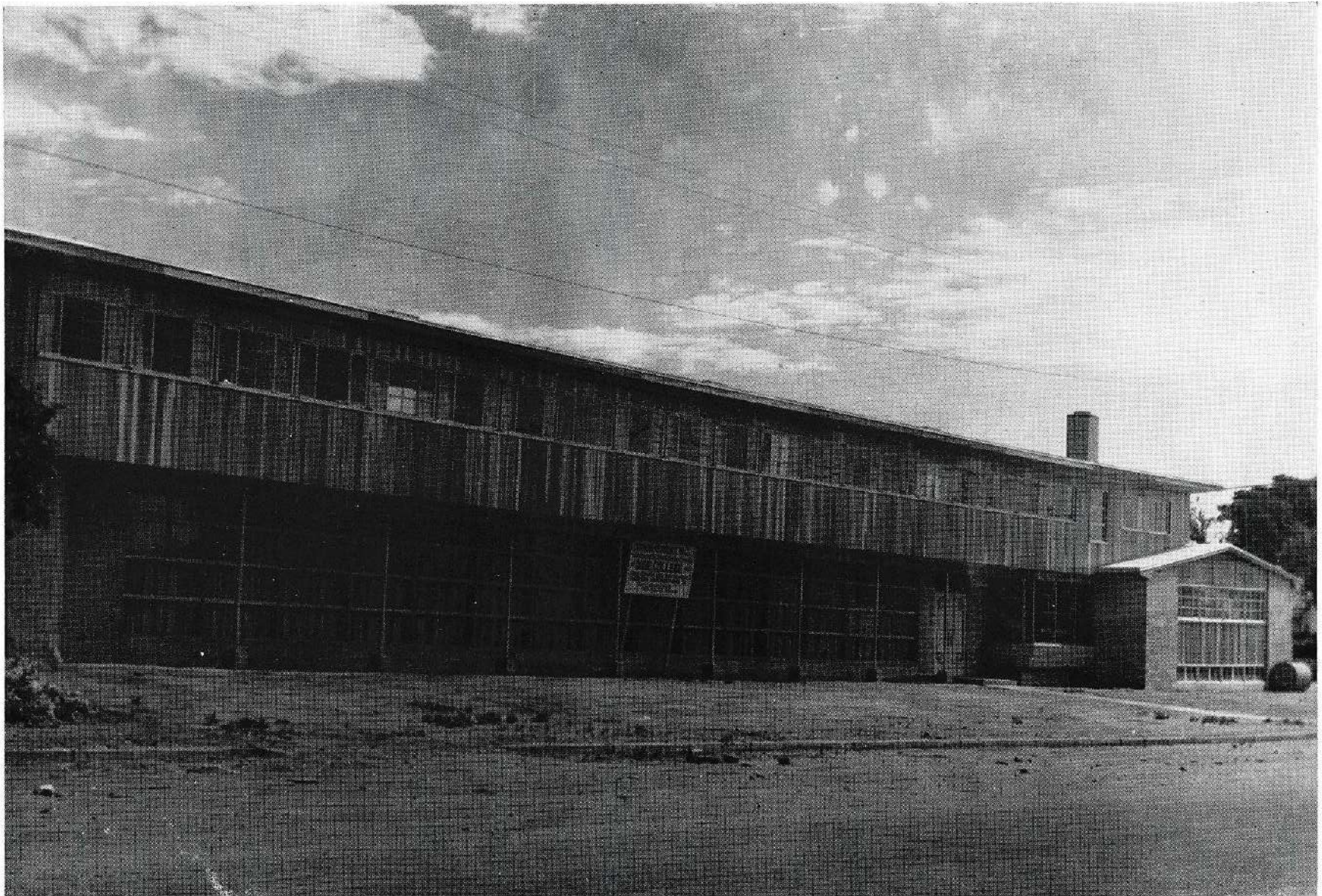
The newly constructed "Dixiana," Dixie College Women's Residence Hall. All proceeds from the 1955 Lions Rodeo were donated to this community project in addition to the individual donations from Lions Club members.
