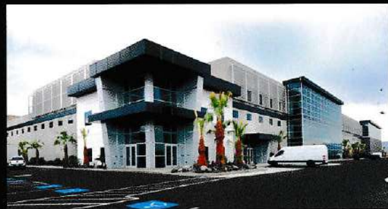
Warehouse / Professional: PAPARAZZI WAREHOUSE Site Area: 12.5 Acres Building Area: 250,400 sq. ft. Completed: June 2021
