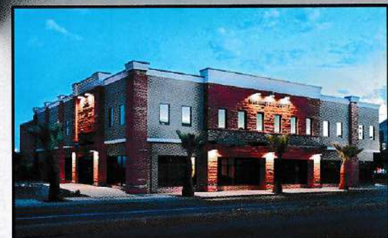
Civic/Education: WASH. COUNTY OFFICE REMODEL Site Area: 1 Acre Building Area: 48,400 sq. ft. Completed: Nov. 2019
