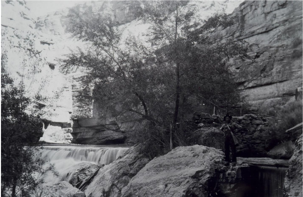
The site for the Dam allowing the river to be diverted into the canal
