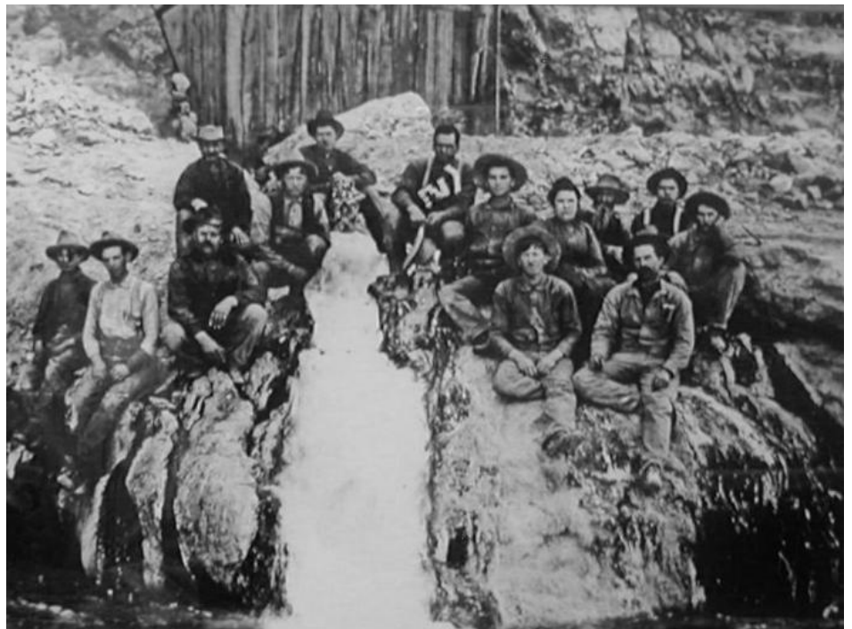
Some of the Canal Workers, Colonists and Miners at the bath house
