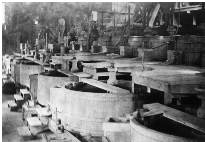
Figure 14. Wooden half-barrels called mullers, in which pulverized ore, water, and reagents were mixed, yielding amalgam of silver and mercury. Silver Reef mining district, approximately 1880, mill unknown. Used by permission, Utah State Historical Society, all rights reserved.
