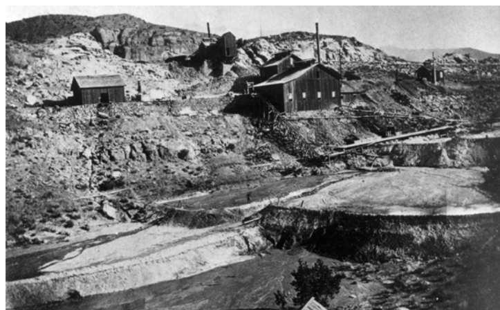
Figure 13. View northwest to the Barbee and Walker mine at White Reef, approximately 1880. Mine hoisting works are in small building at top of reef, above the five-stamp mill. The building on the left is the blacksmith shop and the building on the right is the assay office. Note tailings from mill in foreground. Used by permission, Utah State Historical Society, all rights reserved.
