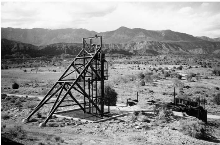
Figure 18. The rebar grate is tremendously versatile. Here a standard grate with concrete grade beam caps the Big Hill shaft. The grate bars are easily fitted around the structural components of the headframe.
