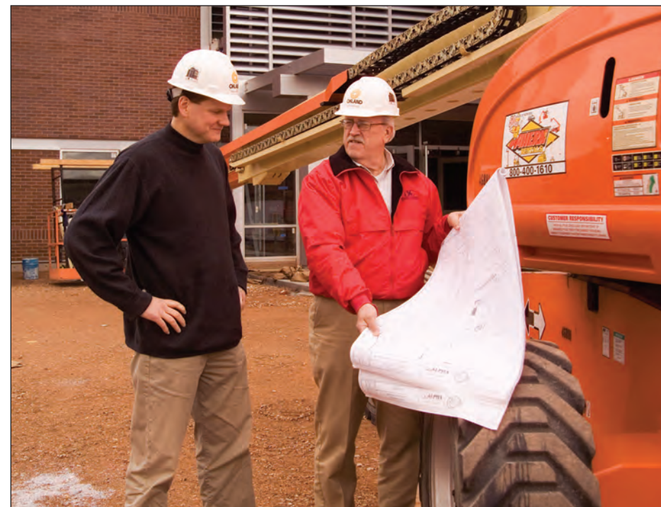
Ned goes over plans with principal architect, Derek Payne, on site of the nearly-completed Russell C. Taylor Health Sciences Building, his last project in his long era overseeing campus growth.
