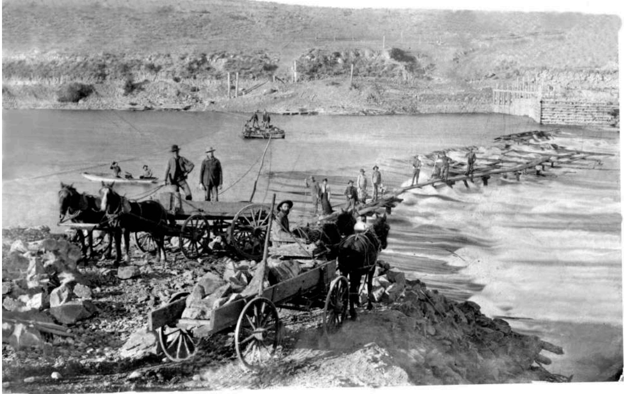
1892 Working on the Washington Fields Dam (1893)
