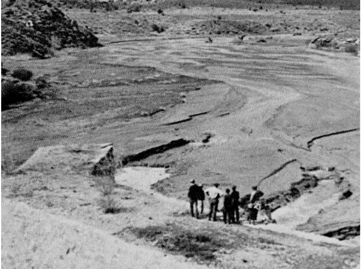
1941 Winsor Dam Upstream Silt Deposits
