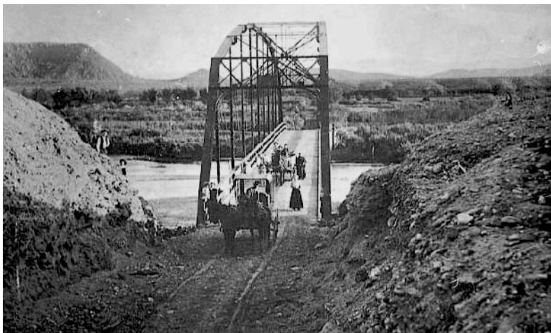
1912 St. George to Washington Fields Steel Bridge over Rio Virgen
