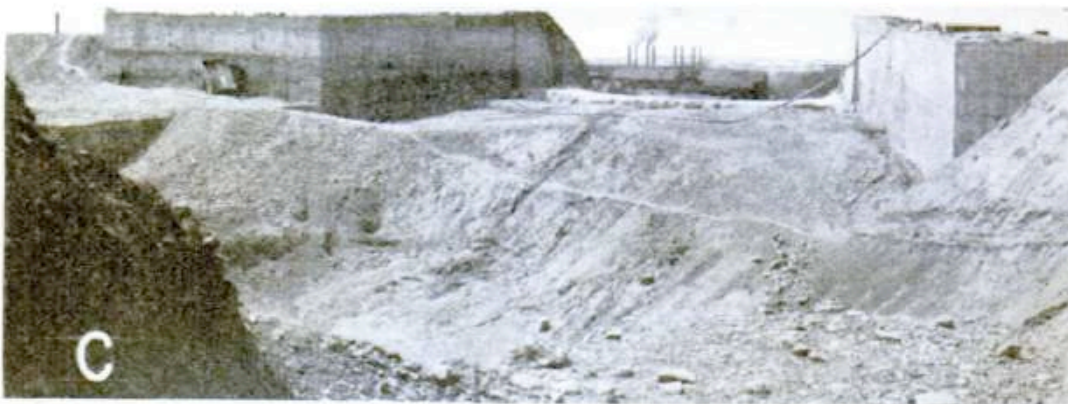
FIGURE 9.—A, Timber and rock spillway, Kanosh Creek, Utah; B, rubble masonry spillway, Willard, Utah; C, spillway with reinforced concrete wings, Kessler Canyon, Utah.
