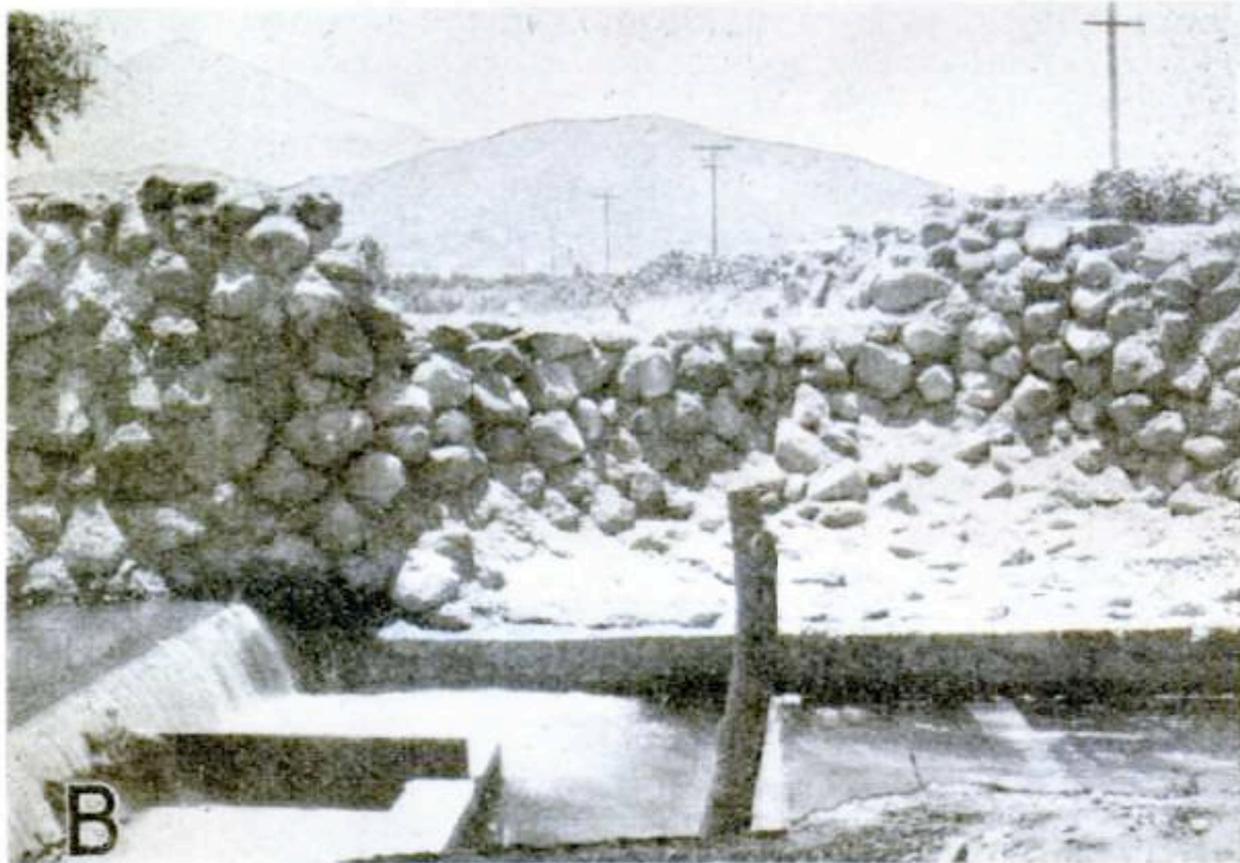
FIGURE 11.— A , Farmington barrier spillway just before being raised in 1931; B , looking upstream through Santaquin barrier spillway--barrier basin lies at one side of low-water channel. Immediately to right of weir crest, placement of boulders in two vertical lines is faulty; elsewhere it is fairly good.
