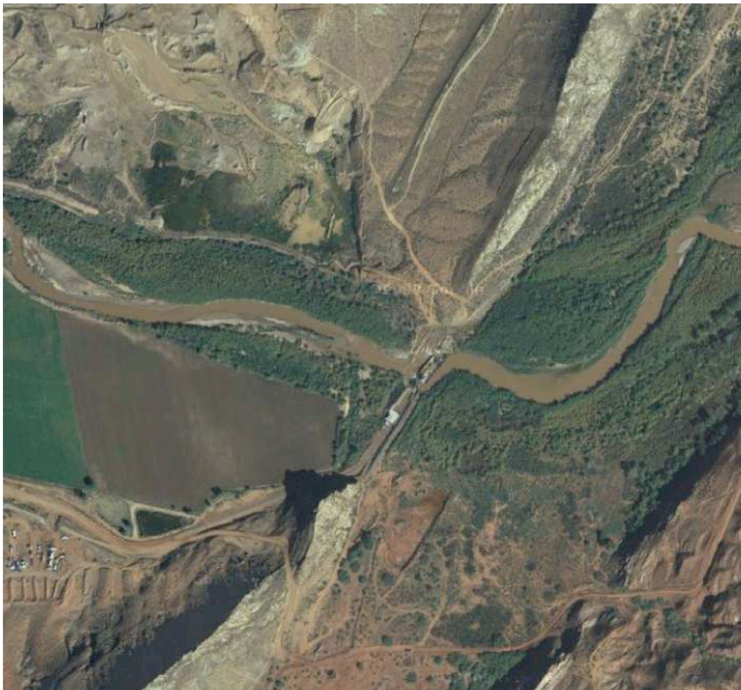
2009 Washington Fields Dam Aerial Photograph
